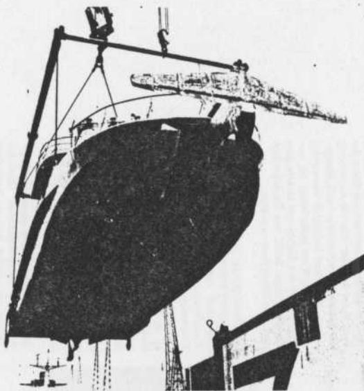
The form of the hull and prow details seen during unloading in Southampton on arrival from the USA. It will be completed in Vosper's Portchester yard.
