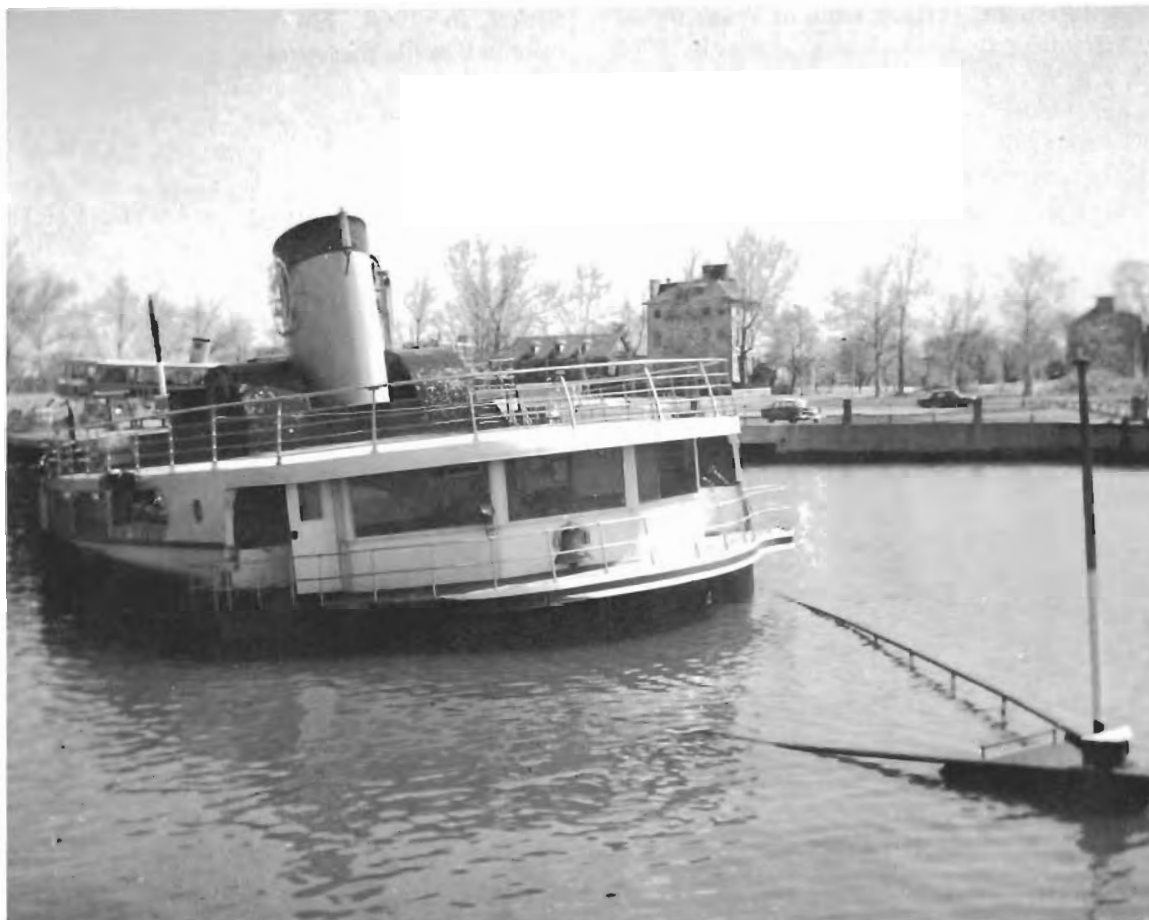
A sight that saddened many Washingtonians: Mount Vernon after she foundered at her Washington pier during the winter of 1963. Peter T. Eisele
