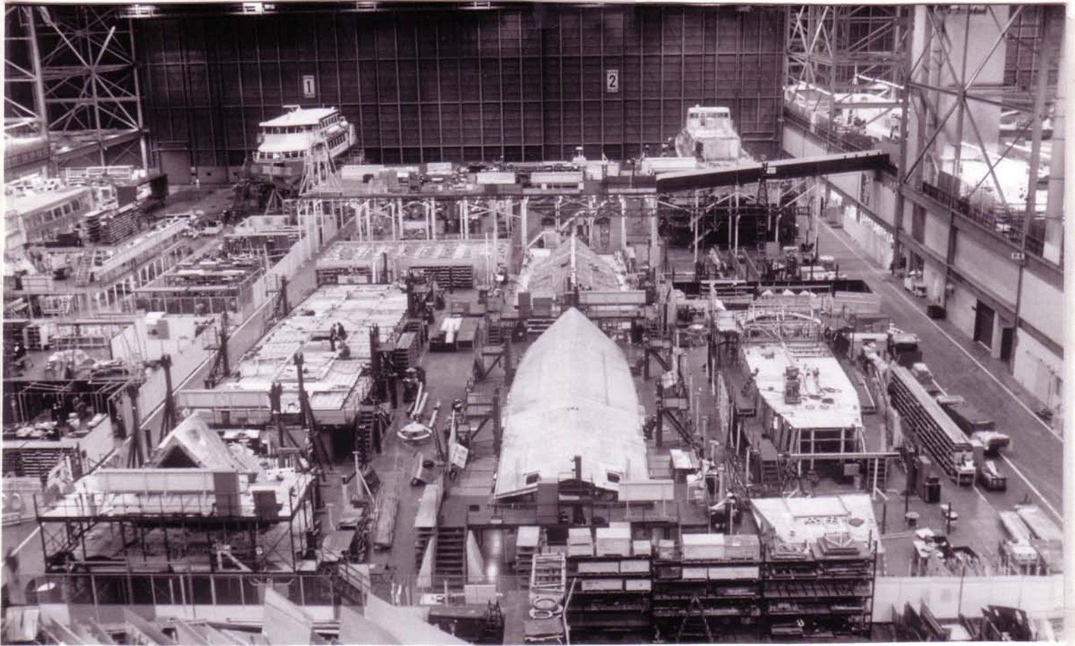
PHM Ships Sub-Assembly Construction (Note JETFOIL In Background)
