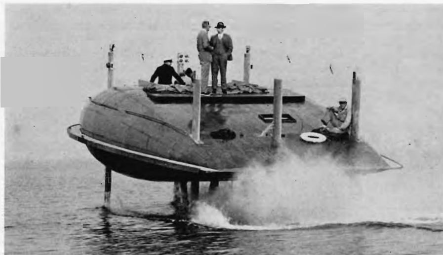
FIG. 19.—NAVY HYDROFOIL CRAFT OF TANDEM SUBMERGED-FOIL TYPE
