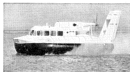
The Westland SRN 5 uses a Gnome engine.
