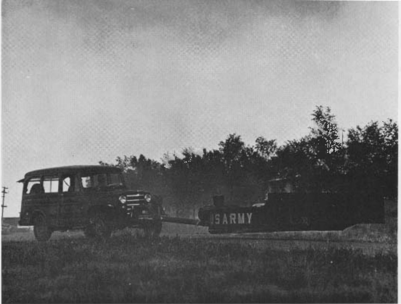
The Frost GEM mine detector carrier. It weighs 800 lb and has a hover height at sea level of 20 in—double the height at which it is seen in this photograph, taken during tests conducted at 10,000 ft above sea level. Photographs by Arnold Gassan
