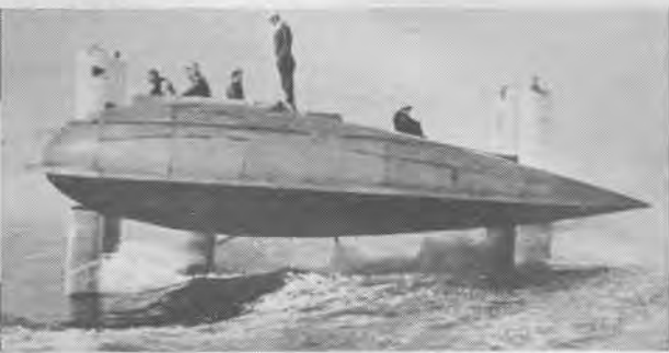
TEARDROP-SHAPED Lantern, Dr. Vannevar Bush's submerged-foil craft of early Fifties, showed stability as passenger rode standing. Foil-control system was ahead of its time.
