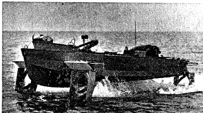
FIG. 22.— 1/4 \cdot 4 SCALE SELF-PROPELLED RADIO-CONTROLLED MODELS OF "BRAS D'OR"
